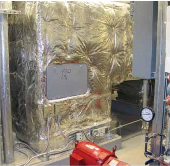
**Figure 2: Proper installation of a combination fire-smoke damper in a duct that penetrates a penthouse floor. The installation has the controller, access panel with an identification number, and indicating lights all in full view and accessible. Photo courtesy of Pat Banse, PE, Smith Seckman Reid.**
