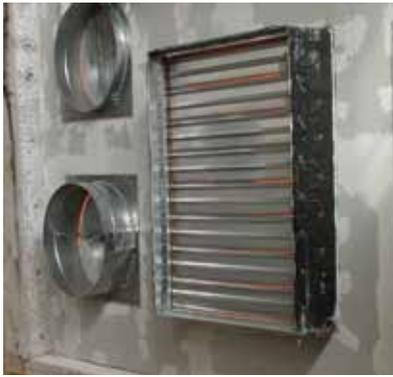
**Figure 5b:** An “out of the wall/partition” fire damper installed on a 2-hour-rated steel/gypsum firewall. Photo courtesy of United Enertech.
