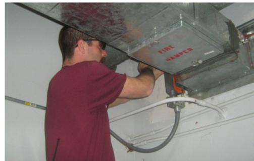
**Figure 2. Placing dampers where staff has clear access saves time and dollars, and it increases the likelihood that all dampers will be found and tested.**
