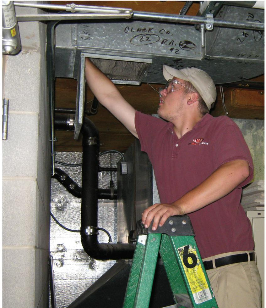
**Figure 1. Accessing dampers for code-required damper inspections and tests increases the risk of hospital-acquired infections.**
