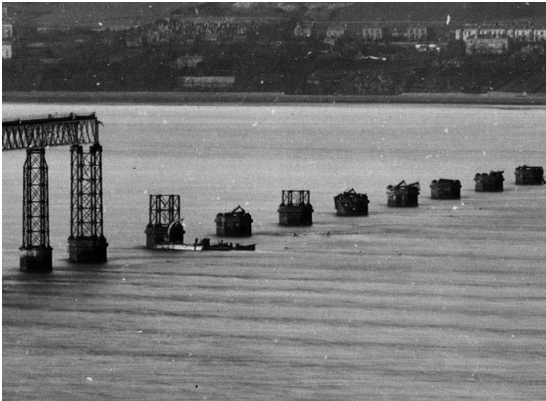
Figure 1 Tay Bridge Failure
