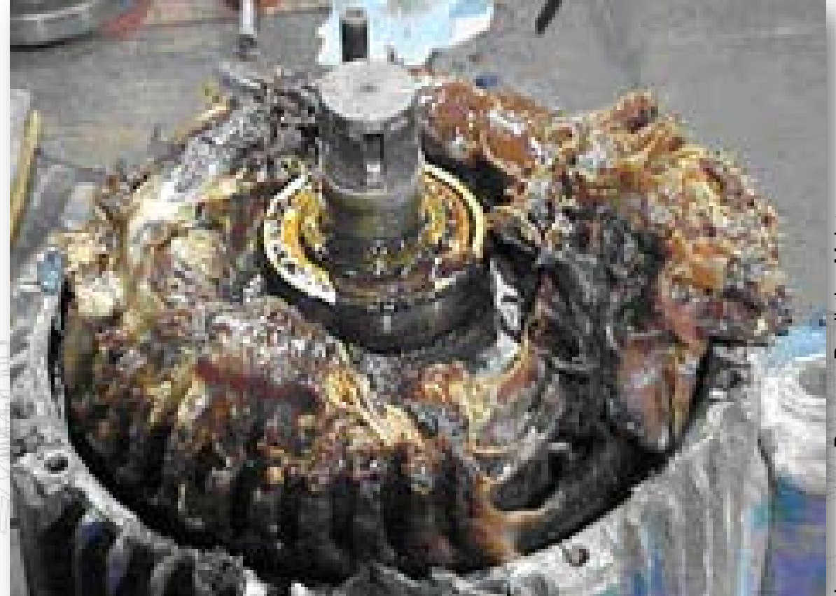
Image courtesy Peterson Predictive Maintenance
