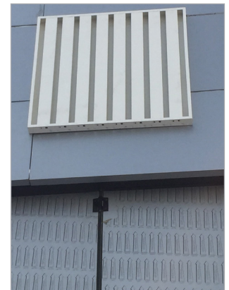
Sand louver with a plate containing holes for sand to exit. Image courtesy of Ruskin Titus Gulf.
