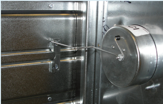
A typical damper position-indicating switch assembly Image courtesy of Greenheck
