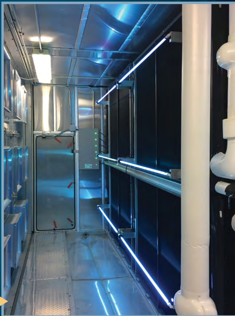
UV lamps installed inside of an air-handling unit.
