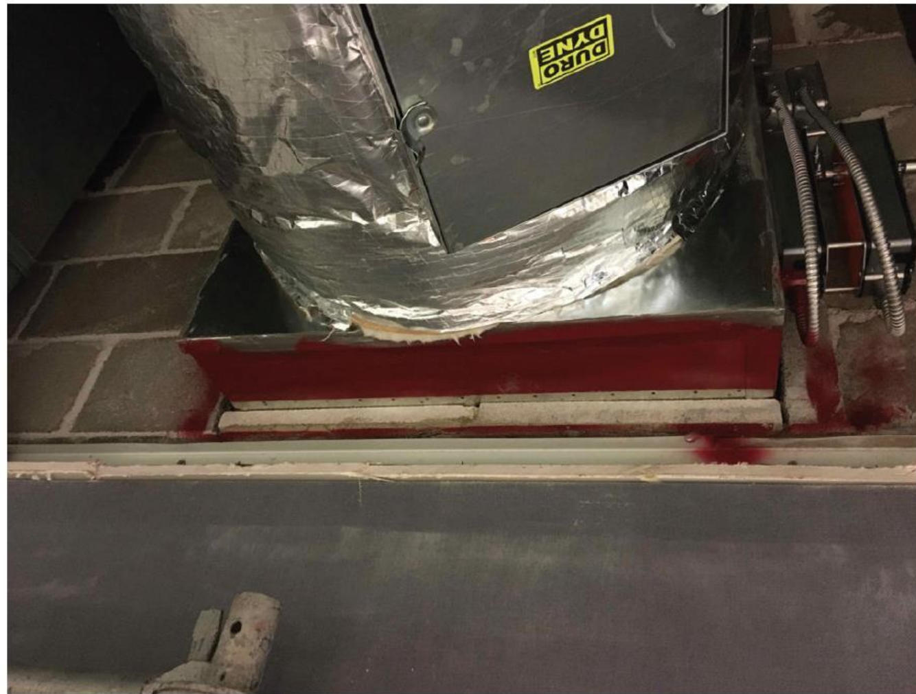
Annular Space Between Damper and Opening
